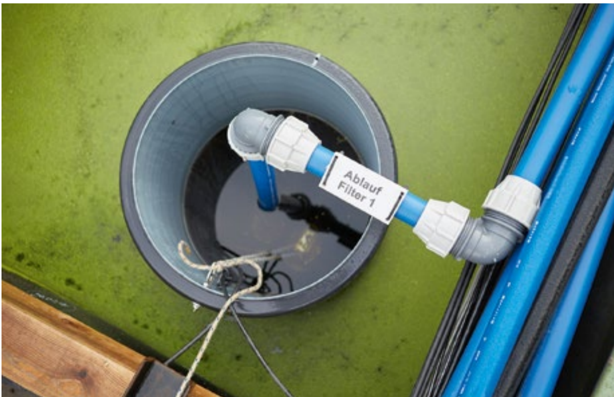
Water drain in one of the filter basins
