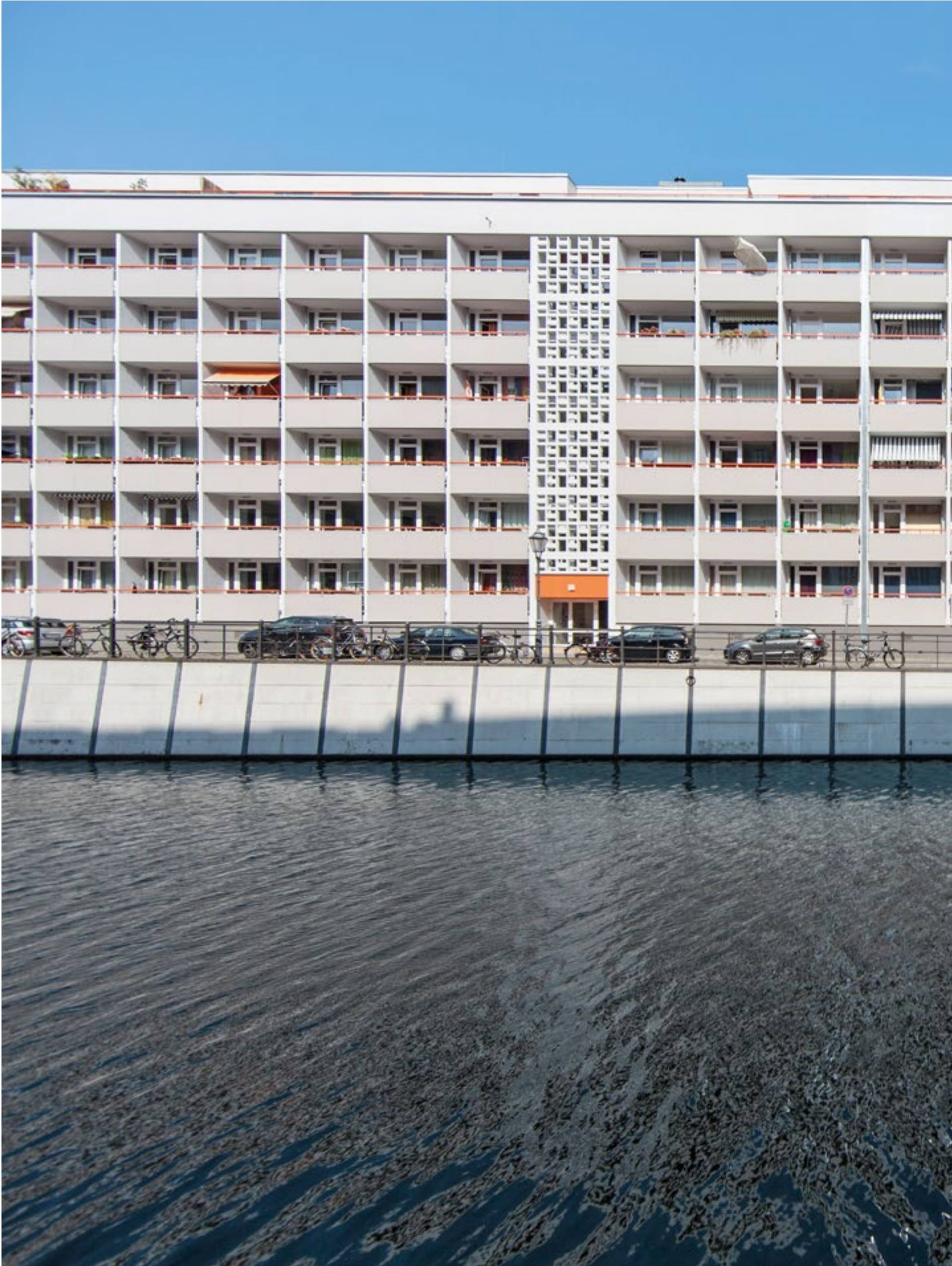
Residential housing at Friedrichsgracht where the future plant filter will clean the Spree water using natural means
